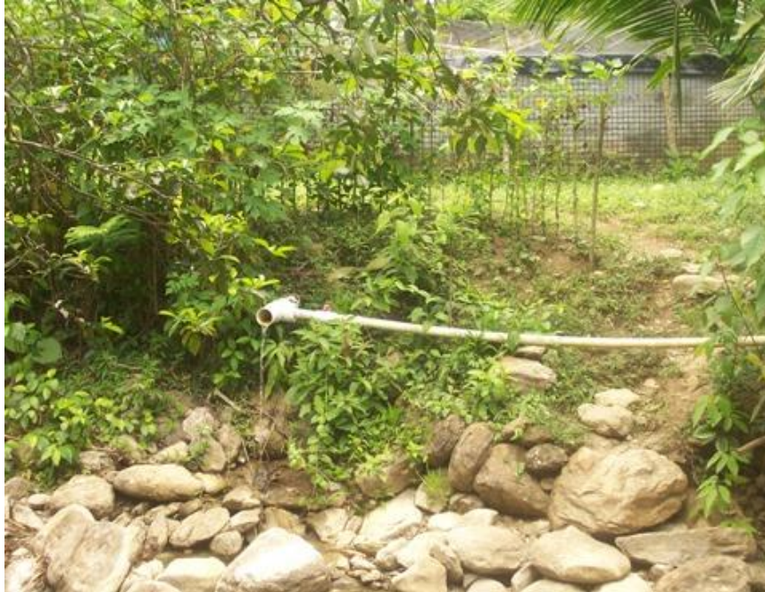
Valve that was used to drain effluent from fish tanks
